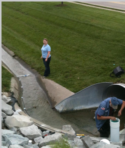
Monitoring stormwater volume and velocity in O'Fallon, IL.
